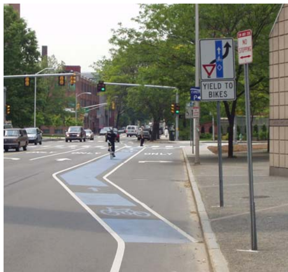
Fig. 2.4E. Blue Bike Lanes – Experimental Marking
