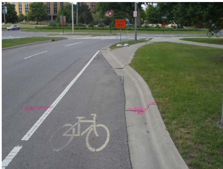
A ramp that eases the transition from a Bike Lane to a Shared-use Path is provided where the Bike Lane ends.
