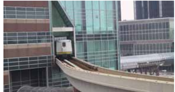
Eight of the 13 People Mover stations are integrated into buildings
