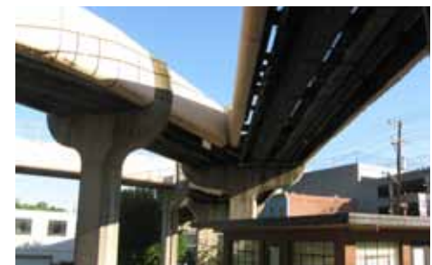
Though portions of the track are at-grade or underground, 65% of the system is built on elevated bridges and viaducts
